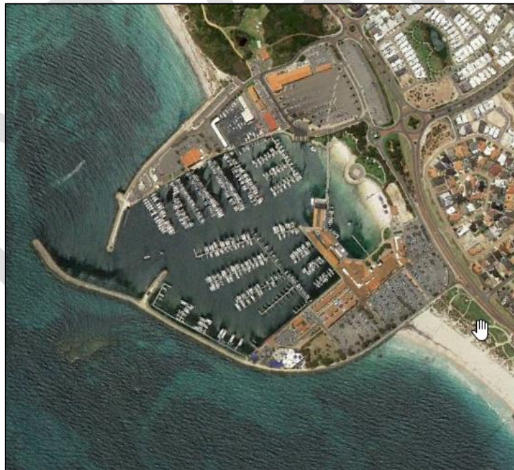
Figure 31. Aerial view of Hillarys Boat Harbour showing berths, pens, stacking facility, shopping precincts, associated apartments and parking.
