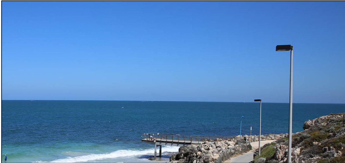
Figure 37. North Beach Jetty (City of Stirling 2019b)
