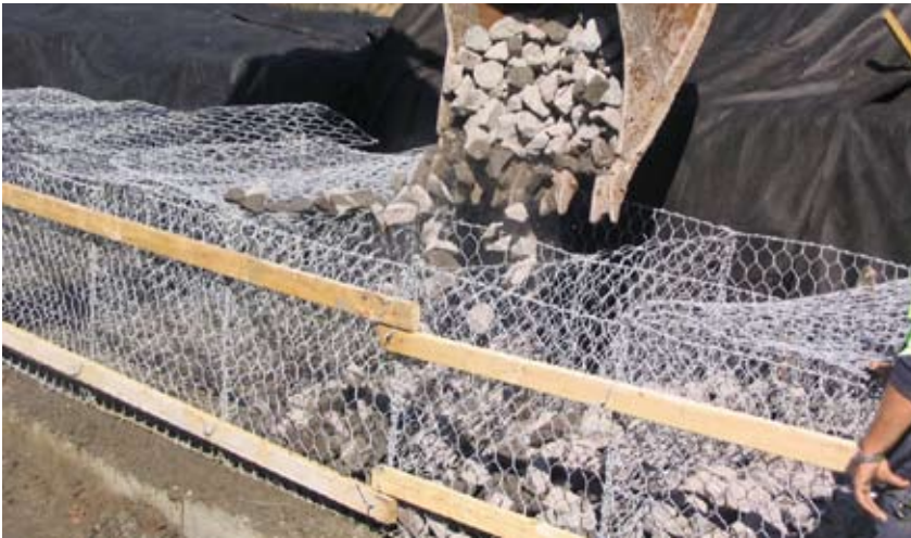
Figure 5.6 Partial filling of gabion units with a hydraulic excavator
