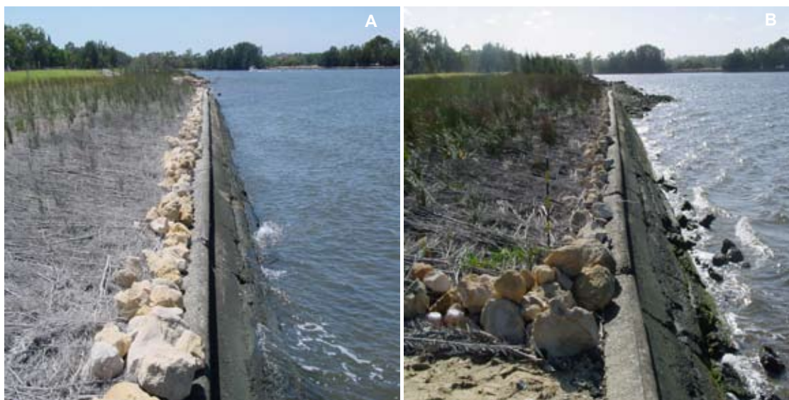
Figure 4.4 Brush matting at Point Fraser above walling
