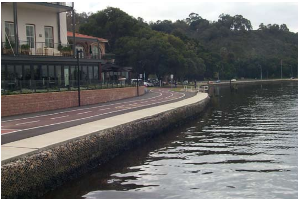
Figure 5.4 Gabion walling adjacent to Swan Brewery development
