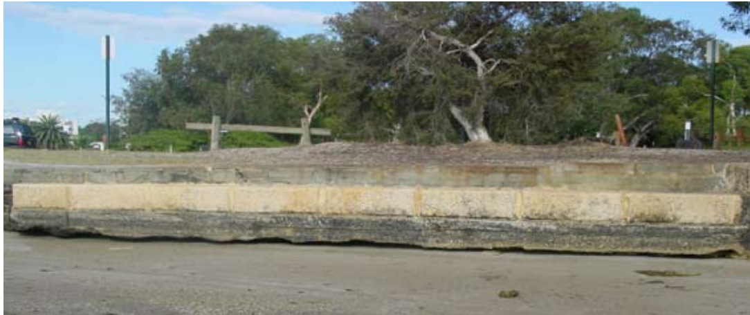
Figure 7.1 Bed elevation lowering in front of a vertical cut block wall – Qantas Boat Ramp
