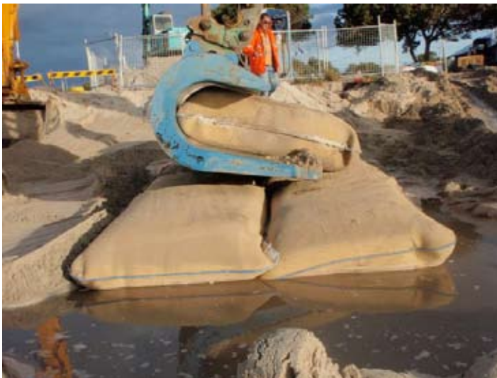
Figure 9.4 Placement of 2.5m 3 geotextile sand container
