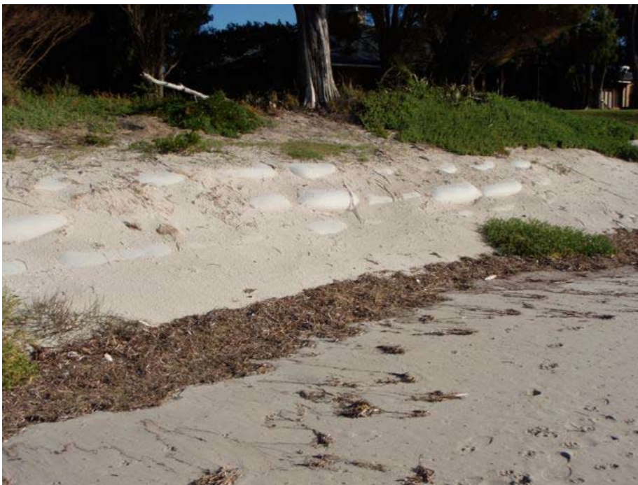
Figure 9.1 Geotextile sand container revetment – Geographe Bay foreshore
