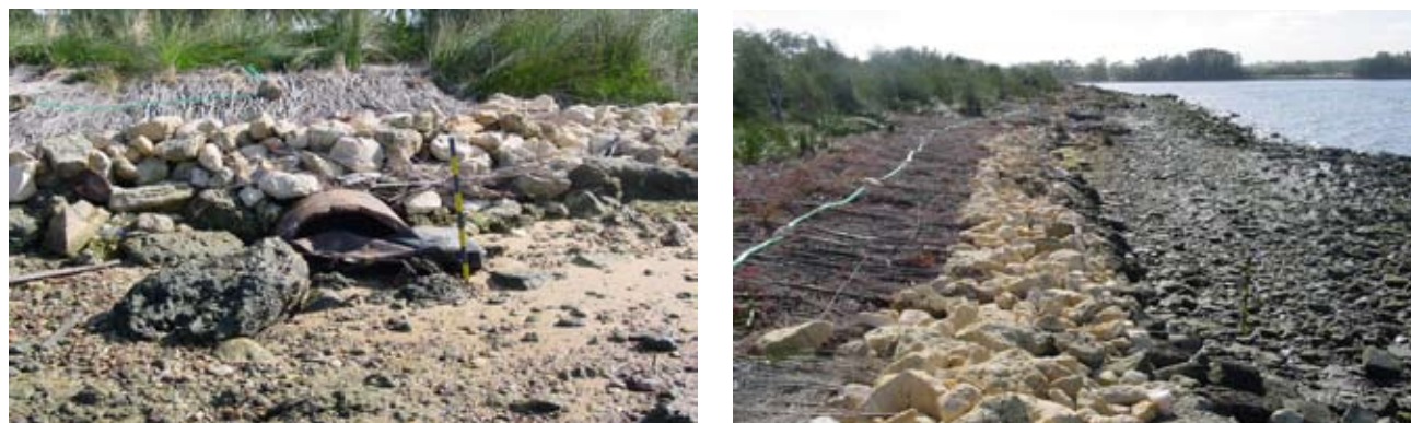
Figure 4.3 Brush matting at Point Fraser with limestone toe
