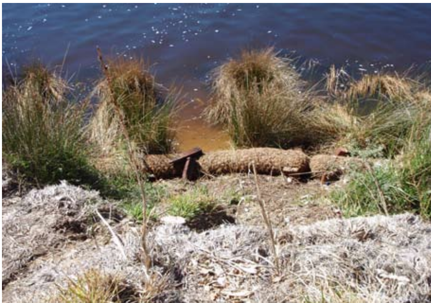
Figure 3.2 Stakes too short
