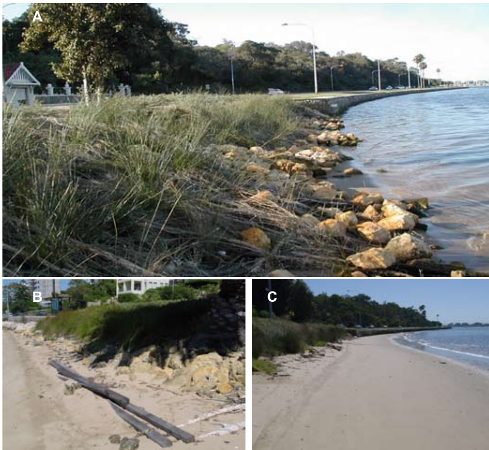
Figure 4.1 Brush matting at Mounts Bay Road
