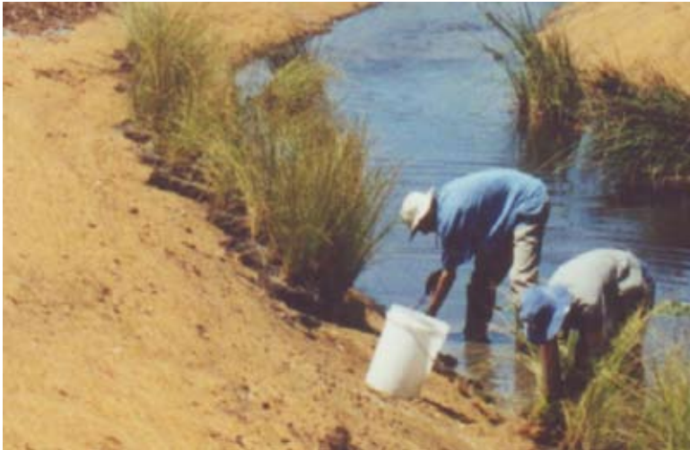
Figure 5.6 Block sedges
