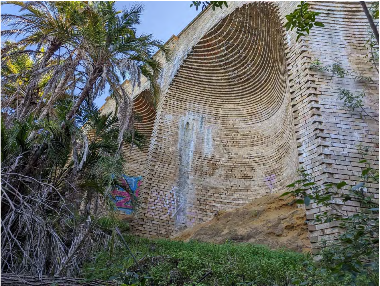
Photograph 3: Arched retaining structure
