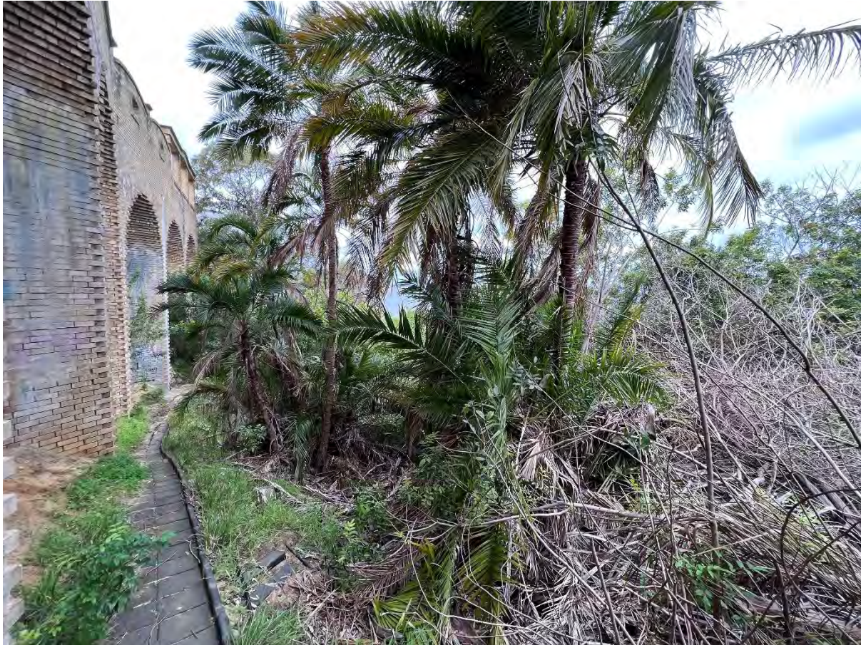
Figure 1 Looking East and Down the Slope from Access Point
