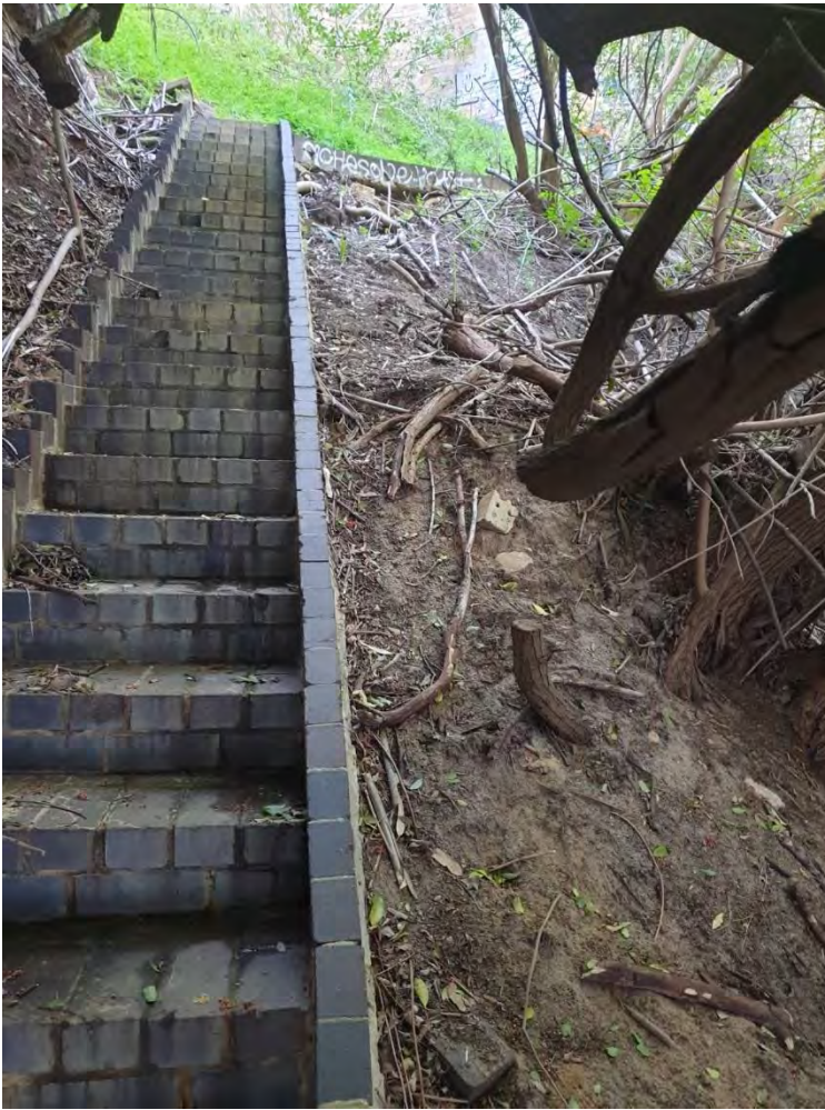
Photograph 2: Masonry steps along the slope
