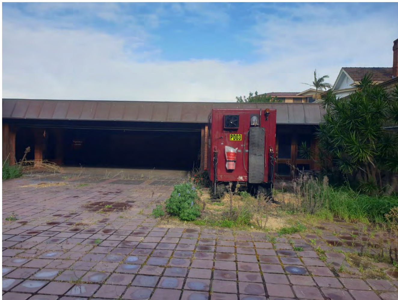
Photograph 1: CPT testing at the residence level
