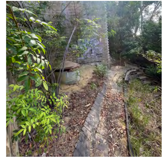
Fig: Bore and degraded walkway
