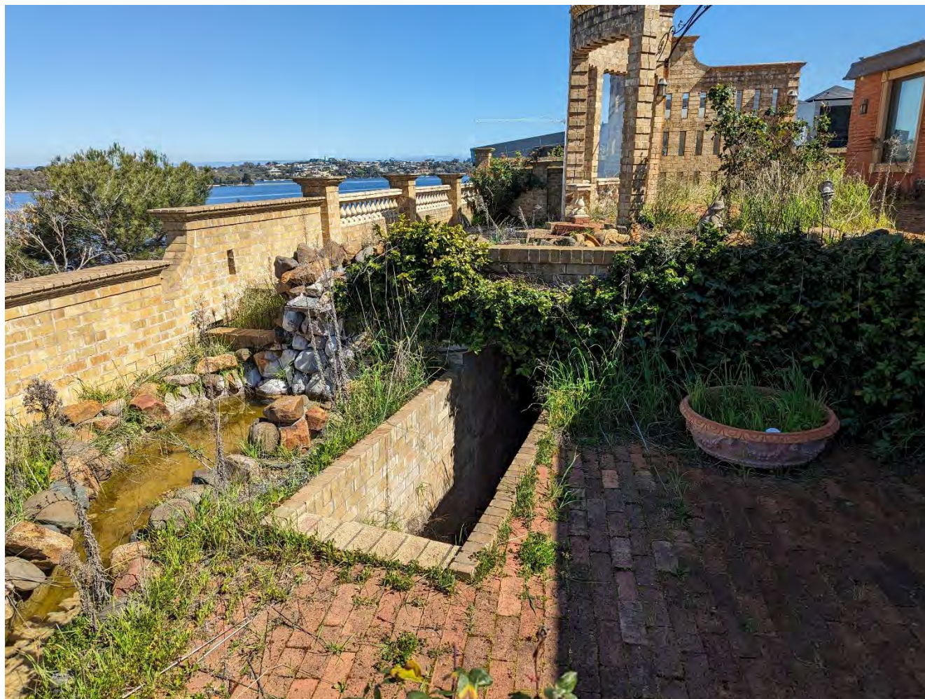
Photograph 4: Looking west at the rear of the residence
