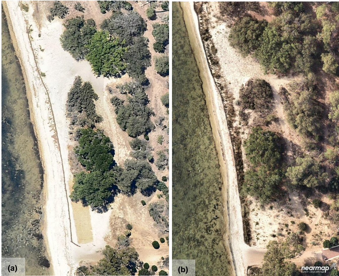
Figure 3 Extent of brushwalling at Point Resolution (north west beach): (a) in early 2015 and (b) in 2020 showing sedge and rush establishment (Source: Nearmap, 2020).
