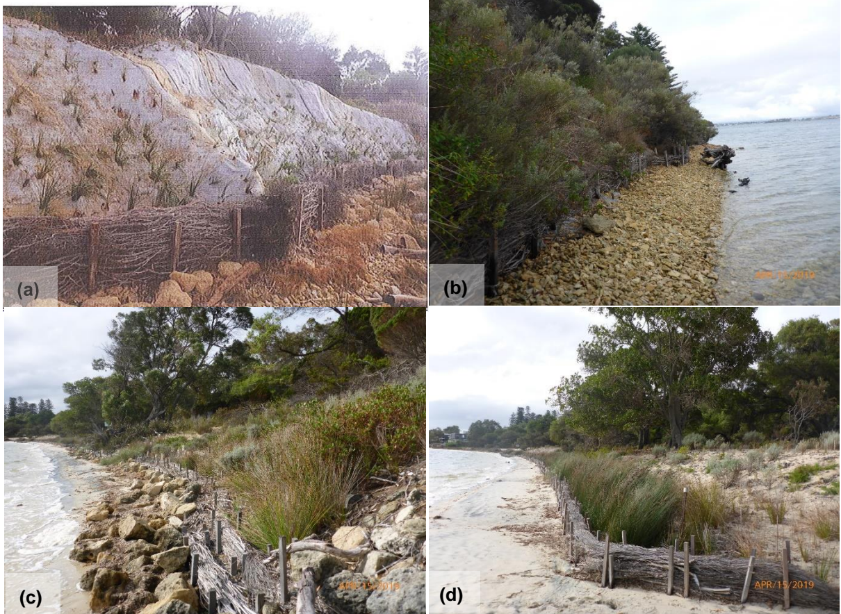
Figure 2 Brushwall use at Point Resolution: (a) against steep slope, (b) the same steep slope 8 years later, (c) double brushwalling for steep banks with high wind wave impact and (d) brushwall without rock rip rap in low impact area 5 years after installation (Source: Syrinx)
