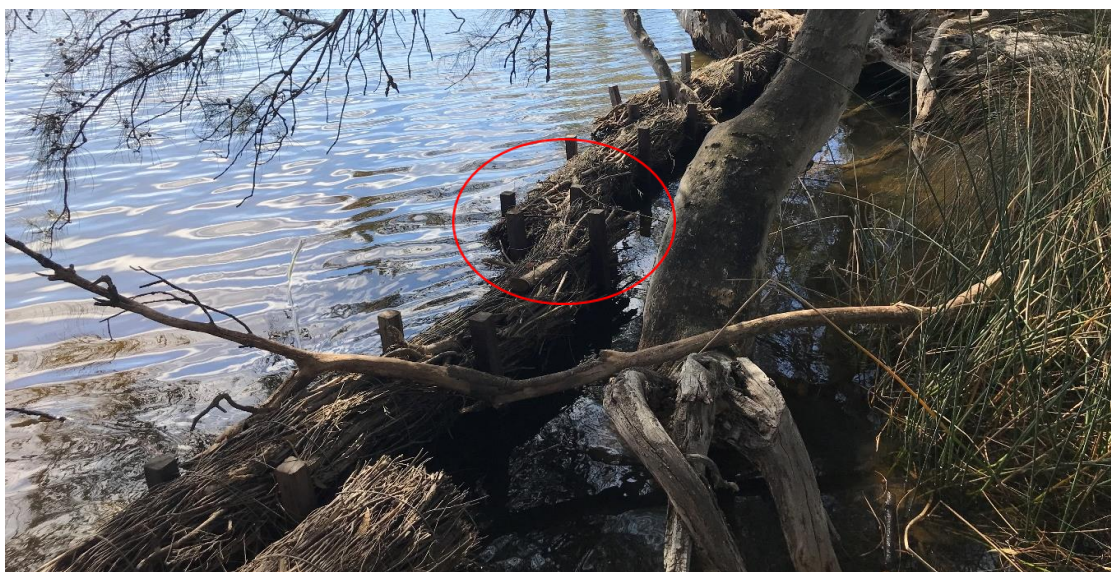
Figure 8 Use of blunt end brush logs with small overlap causing weak points in the brushwall (Source: Syrinx)
