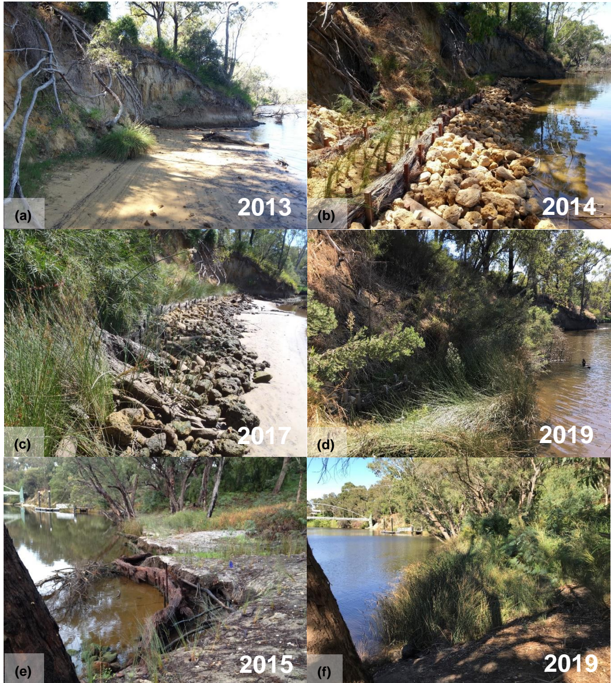
Figure 4 Use of Brushwall to treat erosion at Success Hill Reserve – steep cliffs (a - d) and low elevation scalloped shoreline (e and f) (Source: Syrinx)
