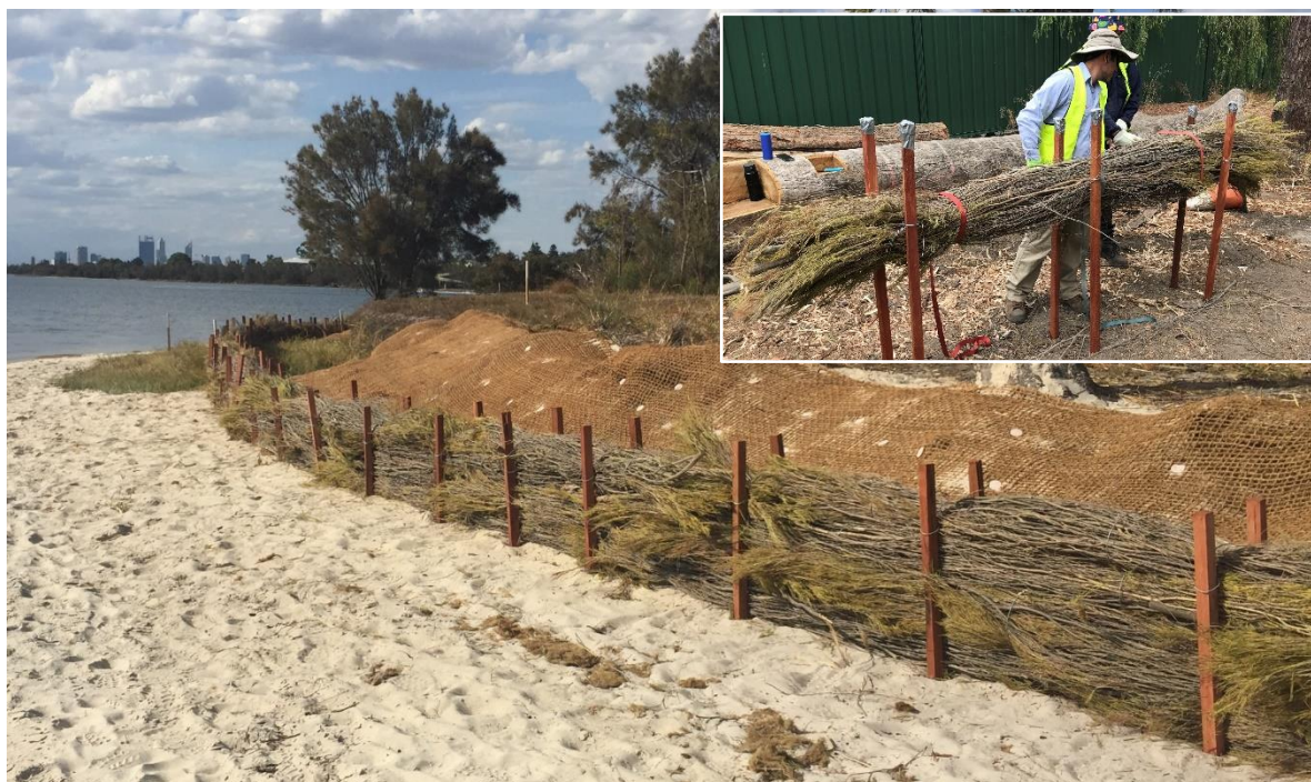
Figure 1 Example of brushwall (main photo) and a brush fabrication (insert) (Source: Syrinx)
