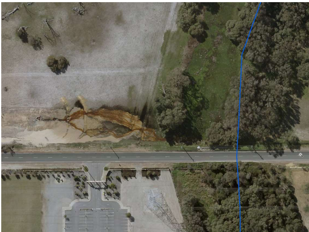
Figure 25: Sediment plume evident on the north side of the Marshall Road crossing.
