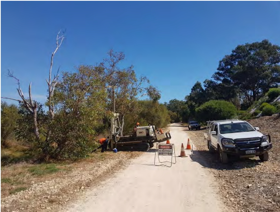
Figure 55: Installation of groundwater monitoring wells MW04D and MW04S.
