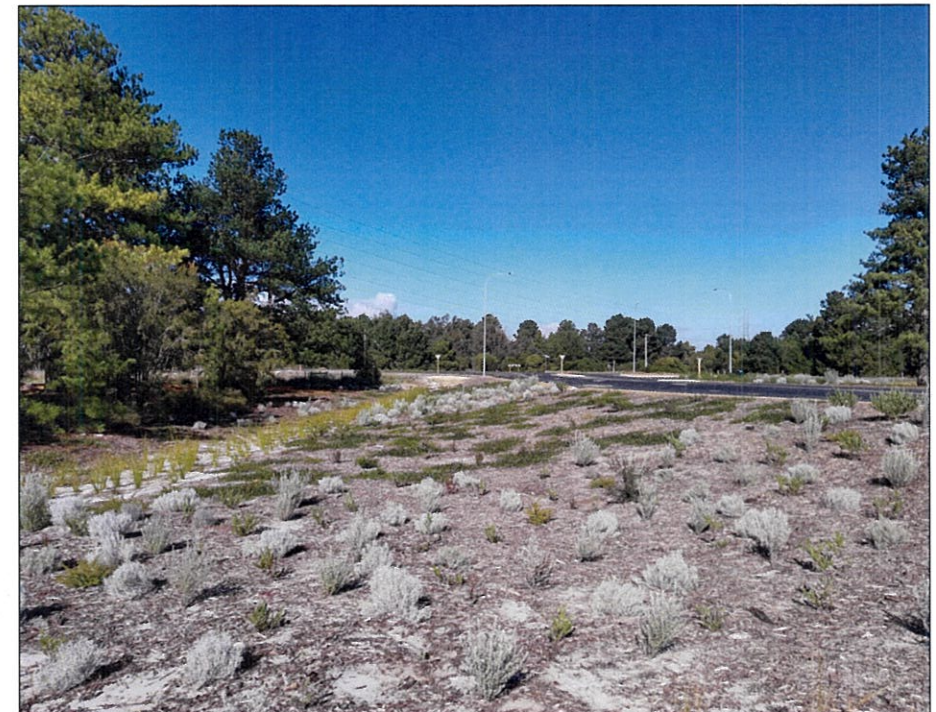
Typical low roadside basin side vegetation to manage fire risk and treat stormwater
