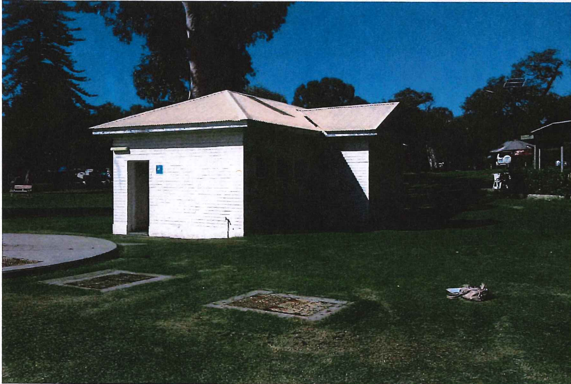
1. Old toilet block to be demolished
