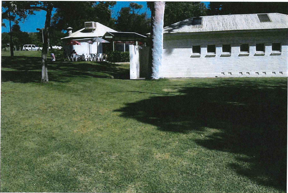
4. View of existing facilities from eastern side where new café will be built
