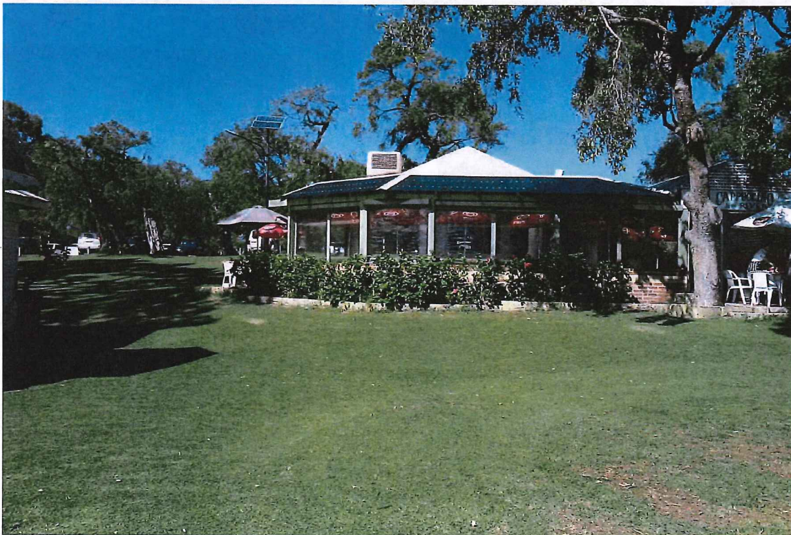
2. Existing café to be demolished
