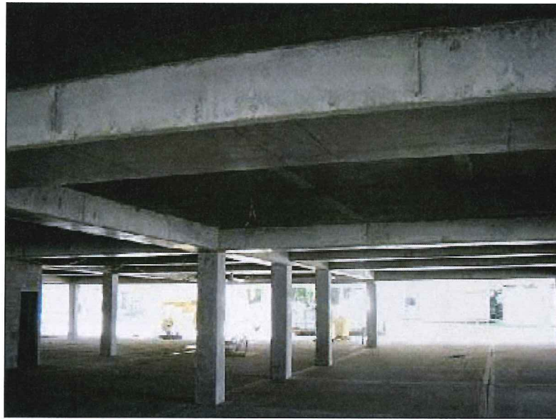
Figure 5. The suspended slab is a design technique often used for heavily loaded structures where excavation options are limited, supported by piers or screw piles.
