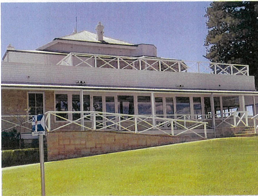
Photograph 02 View from carpark. The main roof form remains, the turret is to be removed and the verandah roof slightly reconfigured. There will be new openings in the store to the left. Griffiths Architects, October 2022
