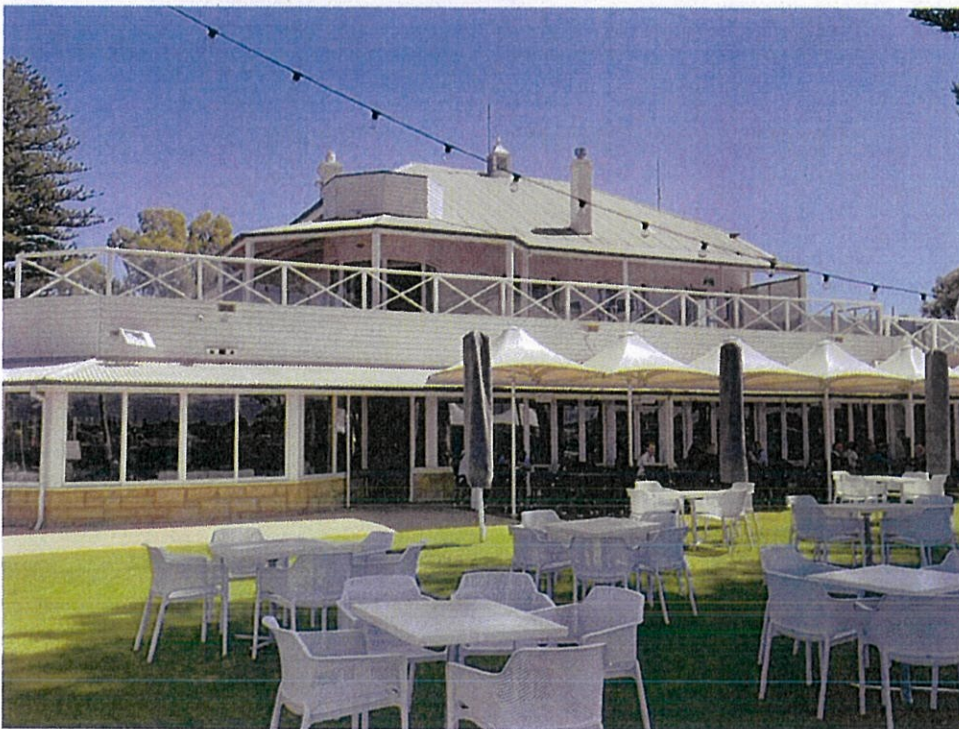
Photograph 04: View from the upper lawn indicating the original roofscape remains the same from this point, then extends west to accommodate the new elements and the verandah roof extends out slightly towards the balustrade. Griffiths Architects, October 2022
