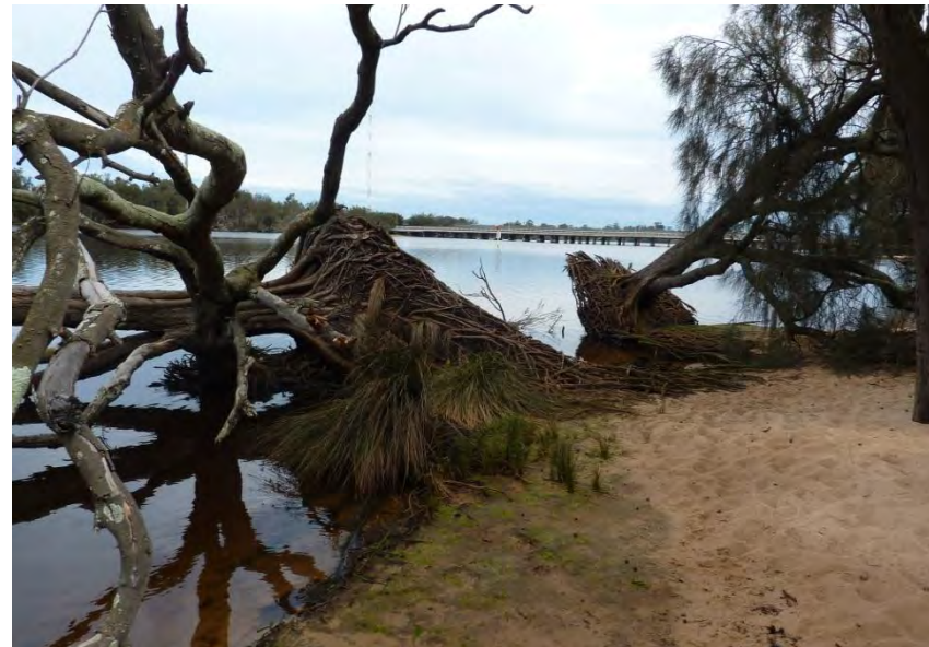
Boat wakes have an impact on tree root systems near Garrett Road Street Bridge. G Pickering
