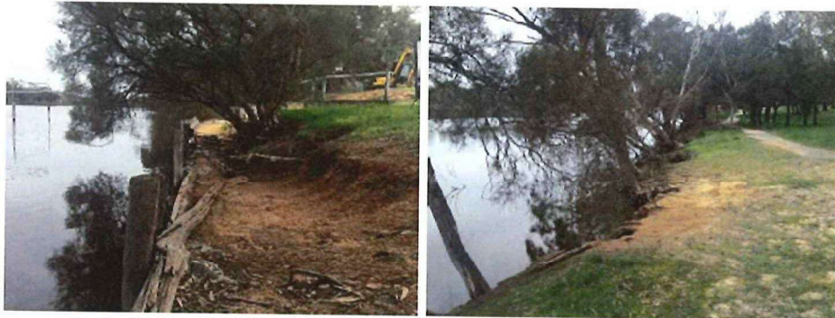
Figure 2.2 Typical Riverbank Condition
