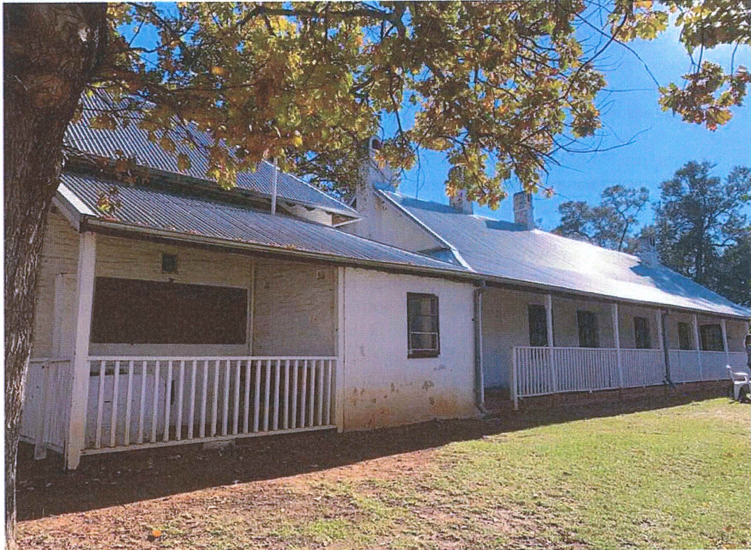
Laundry copper, trough and balustrade to be removed, Main House.
