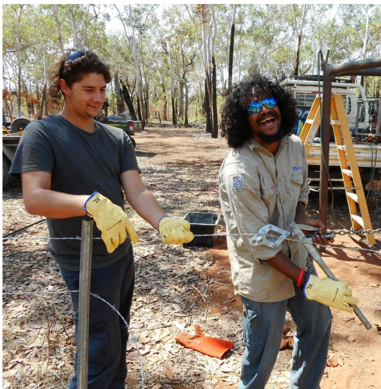
Above: MG Rangers working on a fencing project. Photo - DBCA
