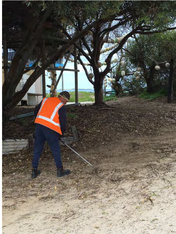
Photo 19. Raking suspected ACM at G115.
