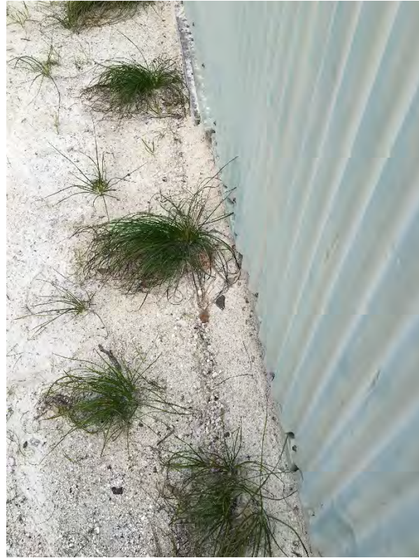
Photo 3. Wedge shack W170, water run off drip line visible in sand where AF samples were collected.
