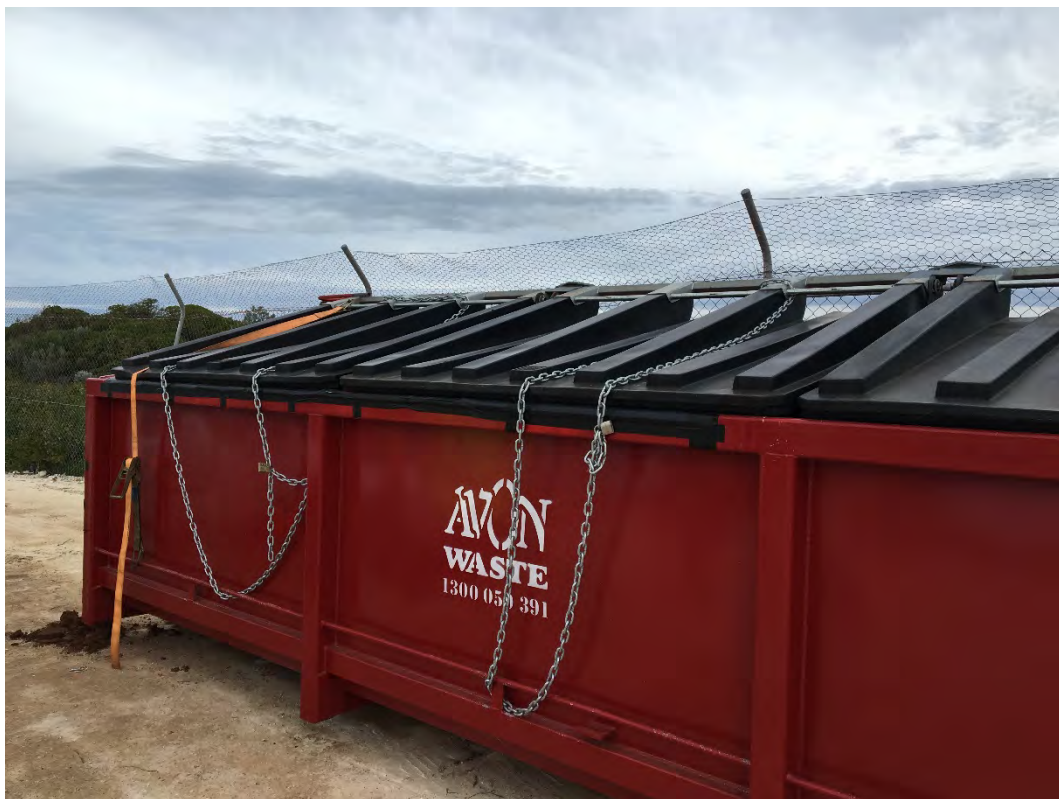
Photo 10. Lockable skip bin for suspect ACM storage prior to its disposal.
