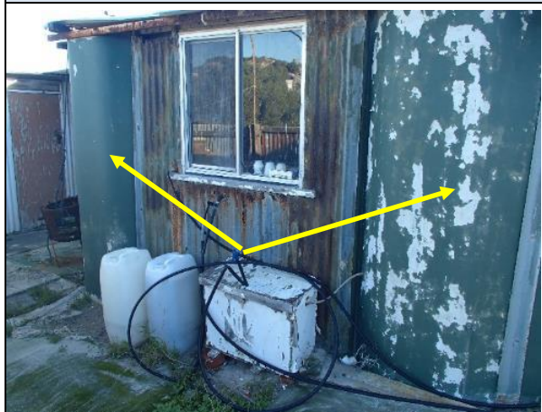
Moulded asbestos cement support columns. Shack G100.
