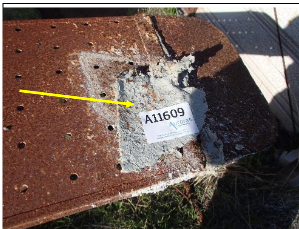
Thermal insulation pad to ironing board, containing chrysotile asbestos. External to Shack W264.
