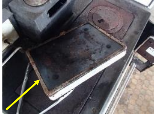
Photograph 12: Bitumen adhesive sound dampener membrane to underside of sink
