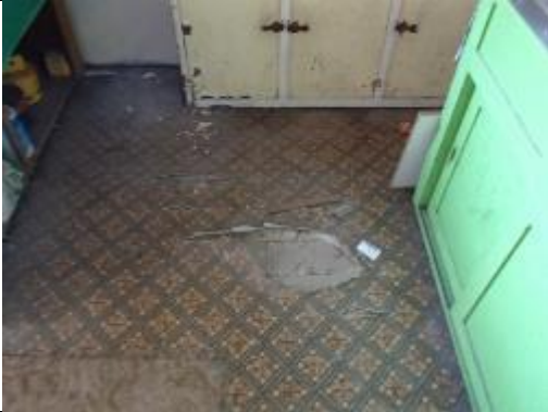
Photograph 11: Loose fibrous membrane material
