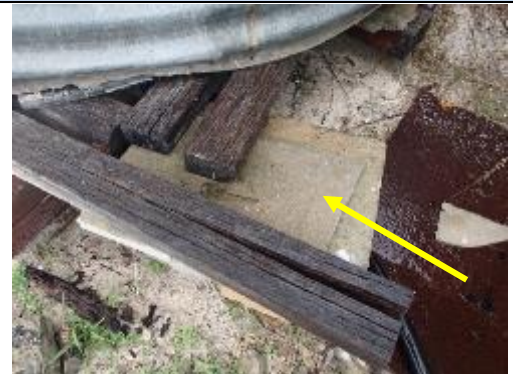
Photograph 14: Cement packers to water tank
