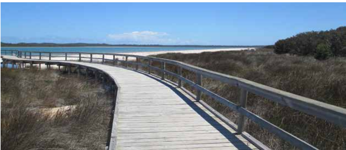
Boardwalk at Lake Clifton. Photo – Grace Patorniti/ Parks and Wildlife
