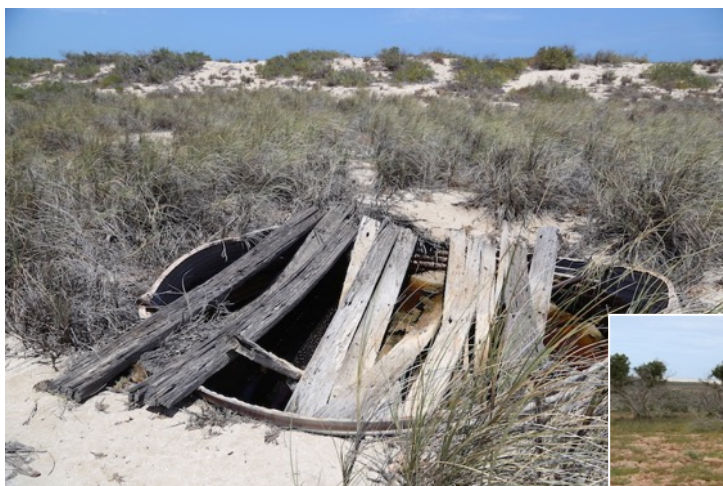
Above Disused well, former Cardabia Station.
