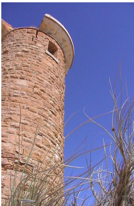
Point Cloates lightstation built in 1910. Photo-Arvid Hogstrom/DBCA
