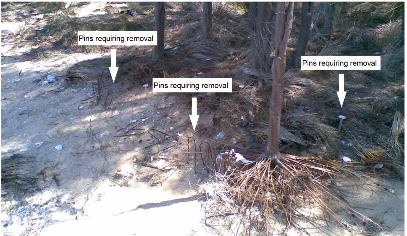
Figure 12 Wire staples and BioGrippers requiring removal after matting has degraded
