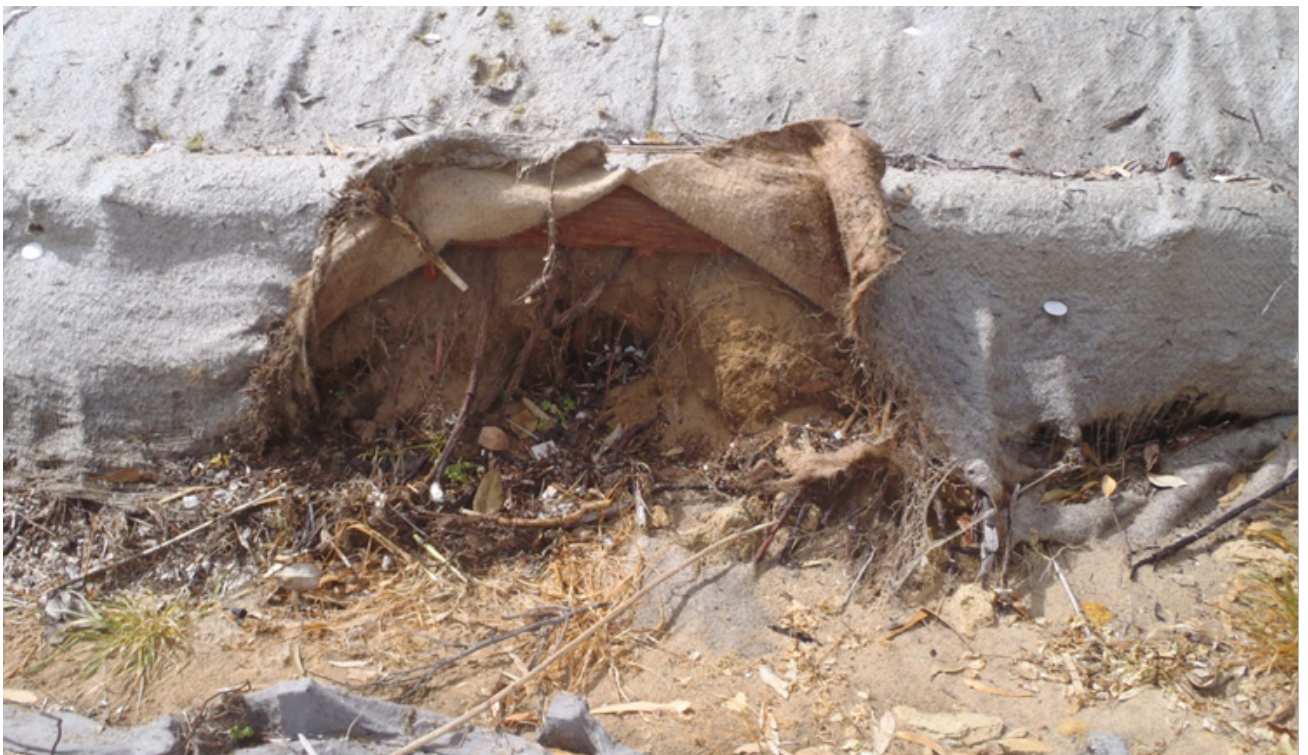
Figure 12 Wire staples and BioGrippers requiring removal after matting has degraded
