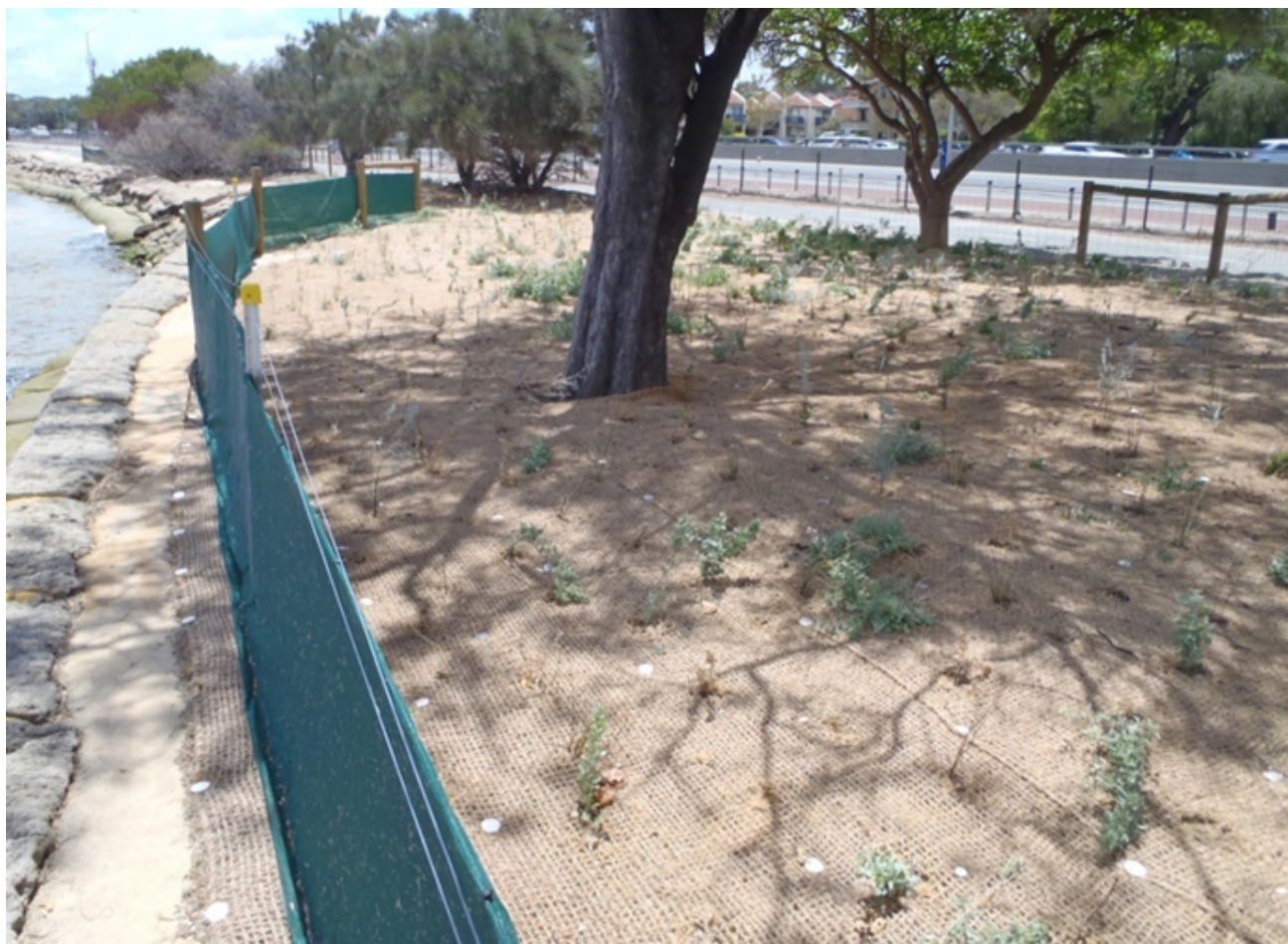
Figure 14 Coir mesh matting, protective fencing and planting. Como foreshore, City of South Perth
