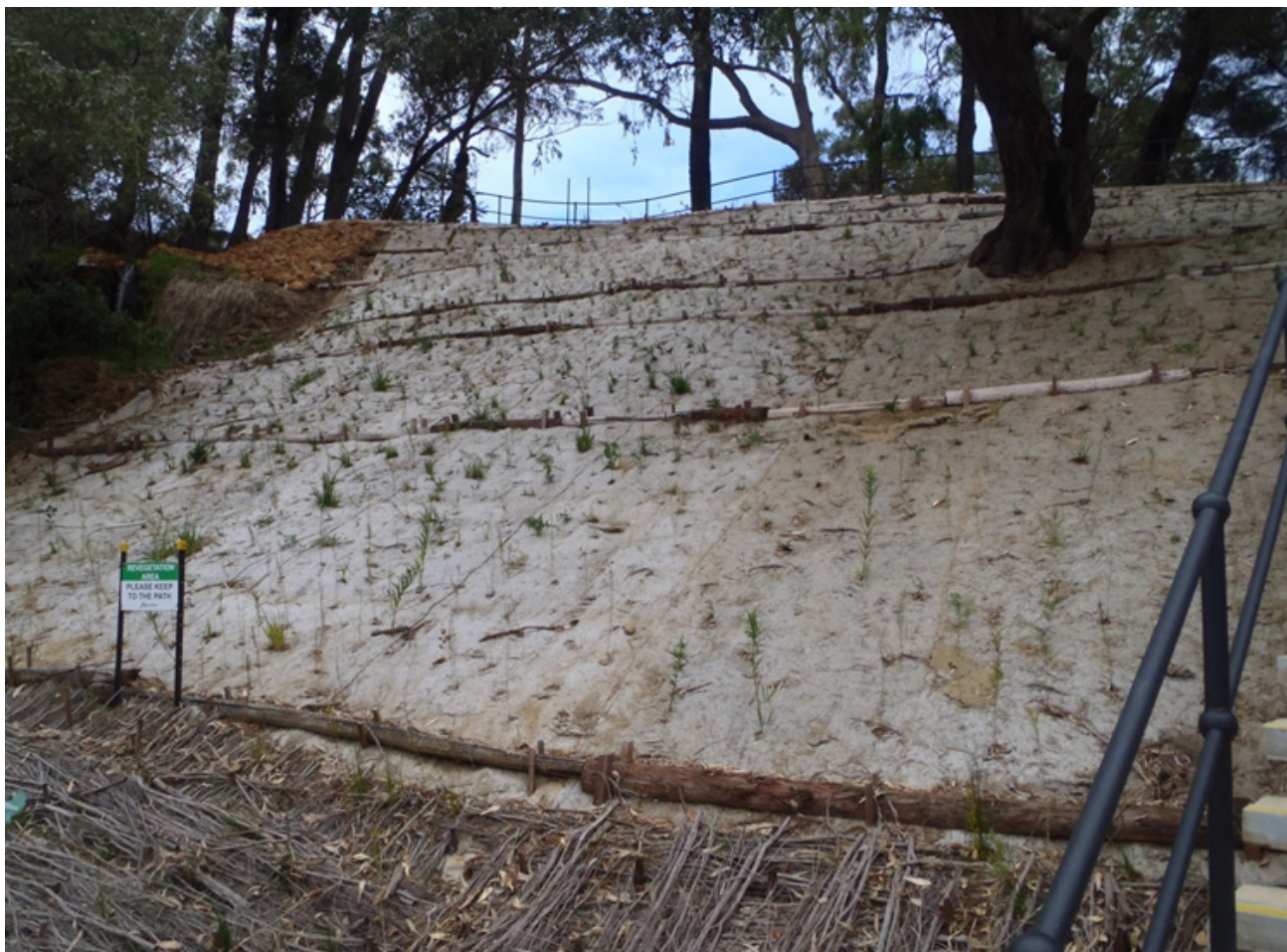
Figure 2 Erosion control matting (jute) and native planting with incorporated bioengineering, Success Hill, Town of Bassendean (Syrinx Environmental, 2012)
