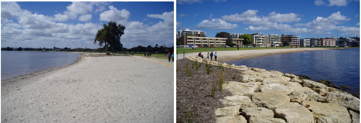
Figure 3.2 Groynes in the lower Swan Canning river system at Sir James Mitchell Park, South Perth
