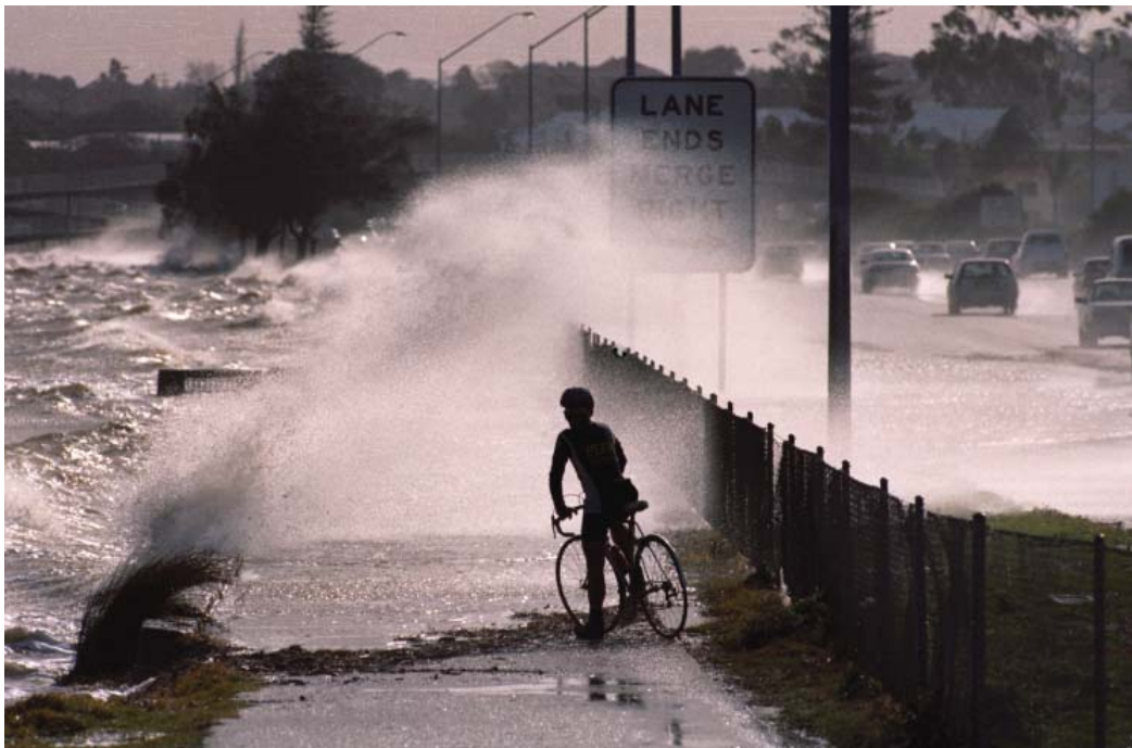
Figure 15 – Waves overtopping a seawall along the Kwinana Freeway during a winter storm in 1995 Source: The West Australian newspaper (13 July 1995)
