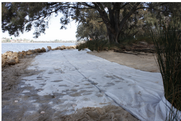
Figure 1 Erosion control matting installed prior to installation of brush mattressing, Prisoners Point (left), and coir mesh used to protect revegetation at a restoration site in the Swan Riverside Regional Park (right)
