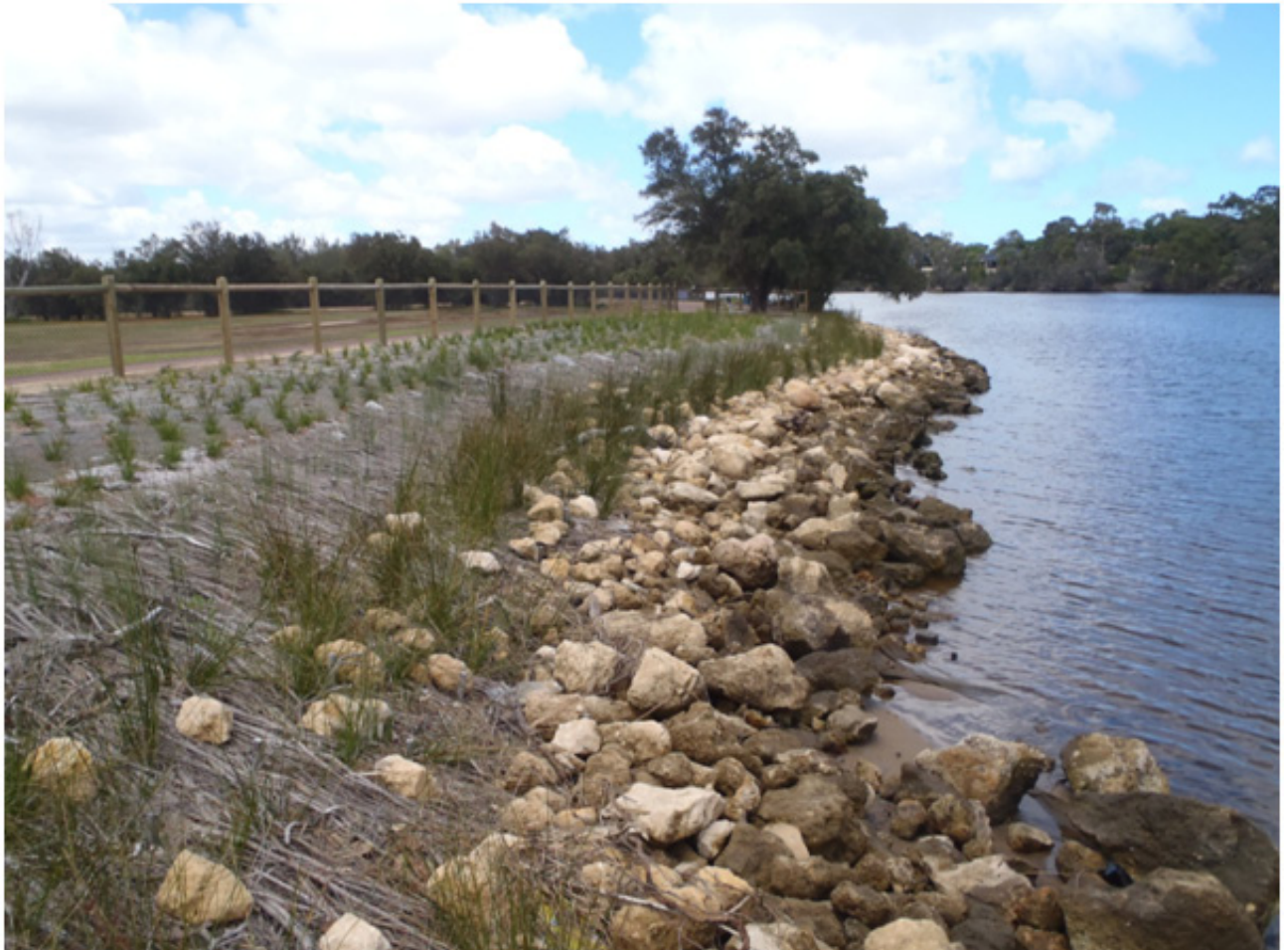
Figure 16 Log brush matting and rip rap, Garvey Park, City of Belmont (Syrinx Environmental PL, 2012)
