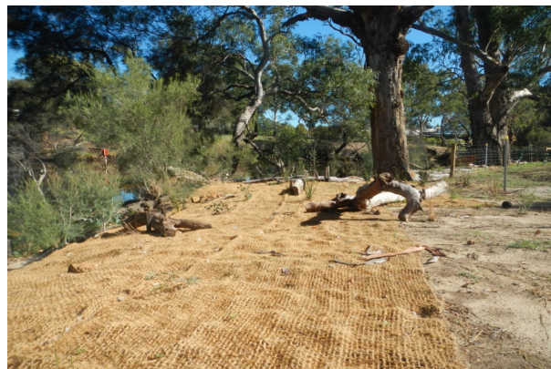
Figure 1 Erosion control matting installed prior to installation of brush mattressing, Prisoners Point (left), and coir mesh used to protect revegetation at a restoration site in the Swan Riverside Regional Park (right)
