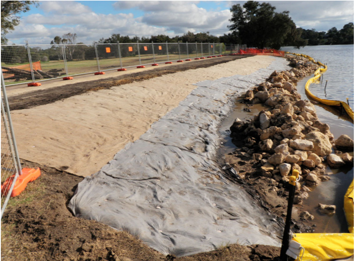
Figure 17 Erosion control matting installed prior to the installation of brush mattresses, Garvey Park, City of Belmont (Syrinx Environmental, 2011)
